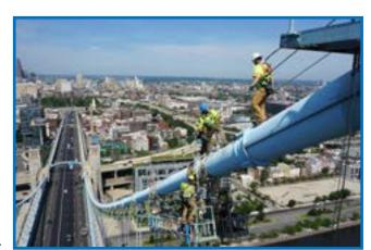
The work also includes repairs to reinforced concrete and steel members, rehabilitation of the north and south walkways, and what will probably be most noticeable to WFS residents, the replacement of the decorative lighting.
